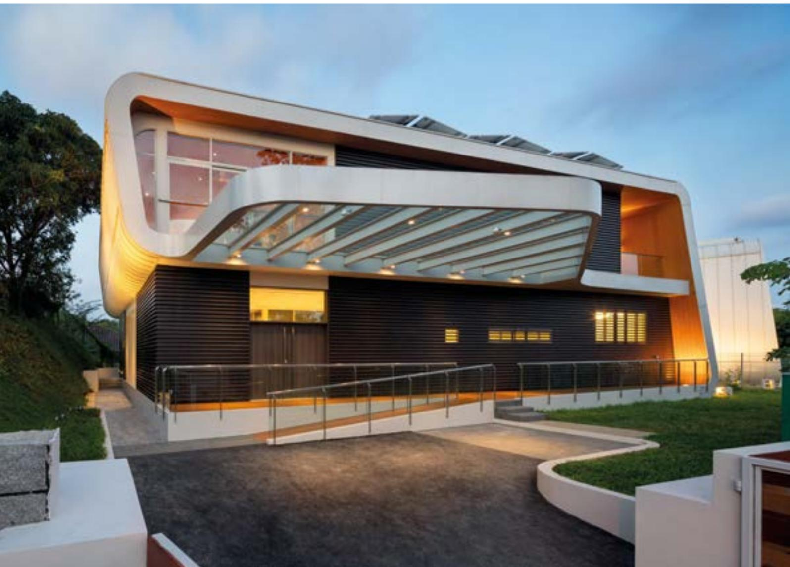
The undulating façade is made up mostly of recycled aluminium and reconstituted timber
